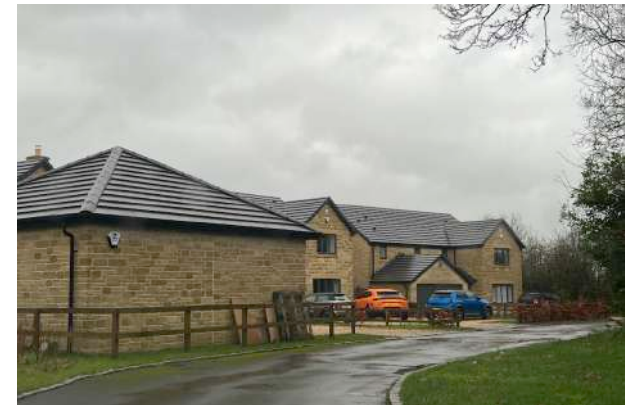
21. New builds on the East of Honey Knob Hill 34a, 34b, 34c and 35 private road
