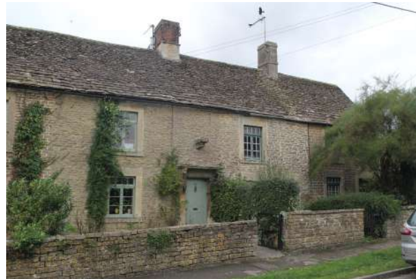
38. Stone tiled roofs on the older buildings. Ashlar details
