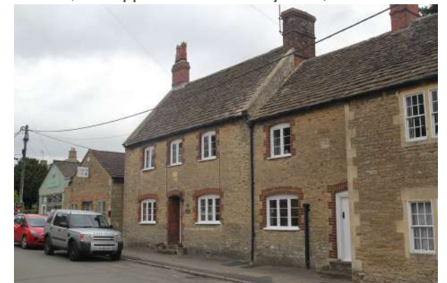
40. Same window and door arrangement of 39, but here bricks are used to detail windows and doors.
