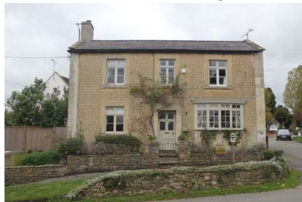
39. As with 38, stone facade and ashlar details as well as the low, flat topped stone wall.
